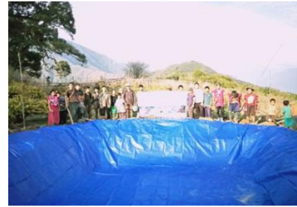
Construction of Jalkund
